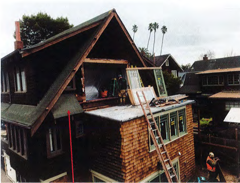
Installation of sliding doors in February 2021
