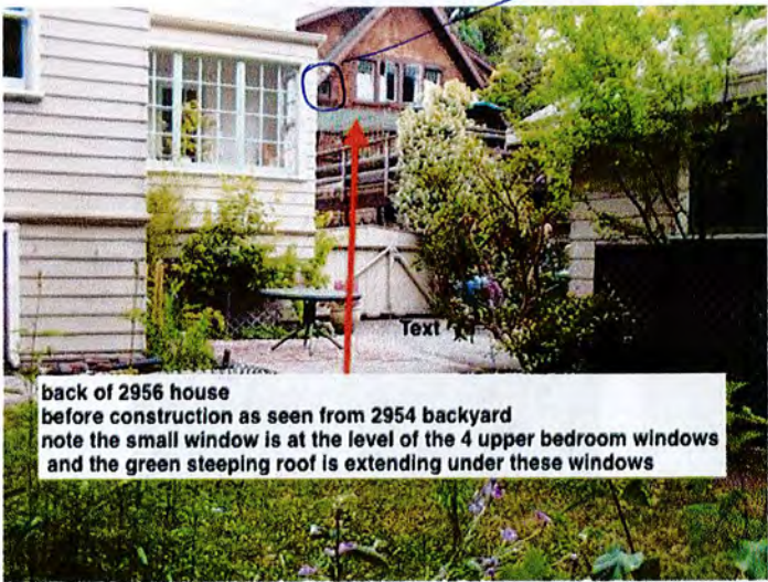
View of green steep roof and 4-pane windows in 2006
